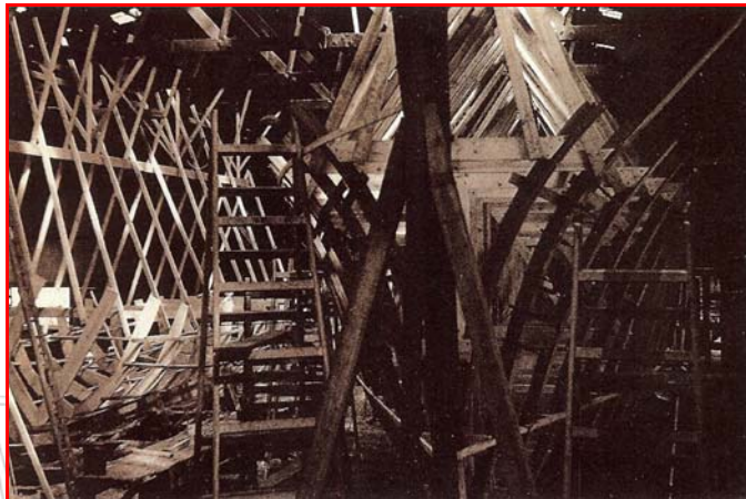
Photograph 62: Maigret being constructed. Note the vertical "A" frame supports which were used in the building of the vessels (© ADMAT Archives).
