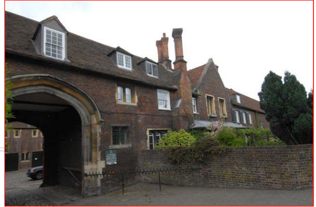
Photograph 25: The front elevation of ADMAT's new office possibly built in 1540 (© ADMAT - Schomberg).
